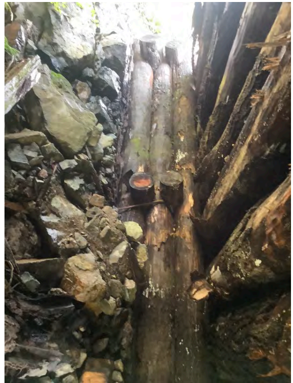
Right Bank Abutment when facing downstream
